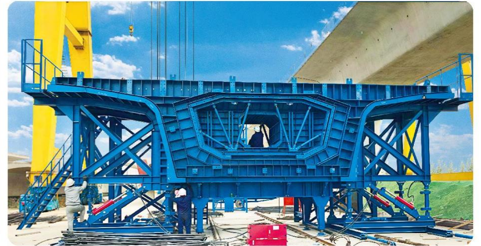
连徐铁路节段模板项目 XUZHOU-LIANYUNGANG HIGH-SPEED RAILWAY PROJECT
