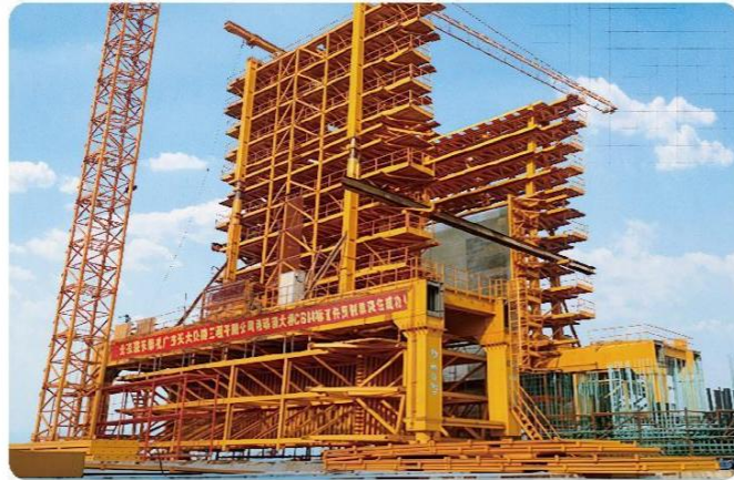
ZHUHAI SECTION CB-04 OF HONG KONG-ZHUHAI-MACAO BRIDGE
