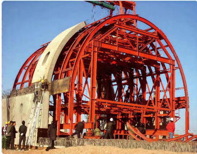
兰新铁路项目(防风隧道) LANZHOU-XINJIANG RAILWAY (WINDBREAK TUNNEL)
