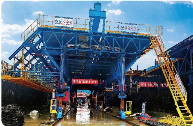
TAIHU LAKE TUNNEL REBAR BENDING PLATFORM PROJECT
